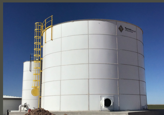
Potable Water Tank
